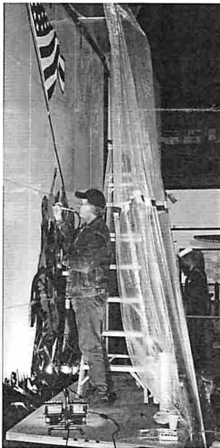
Mike Weinbrecht repairs the damaged porcelain area
