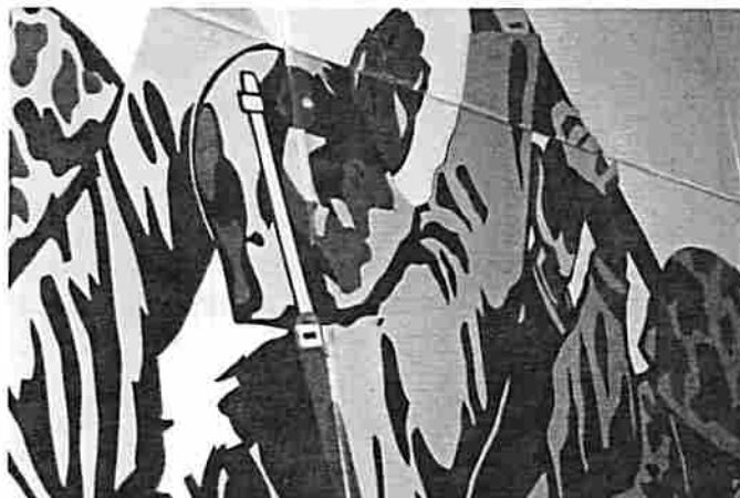
Detail of the finished repair
